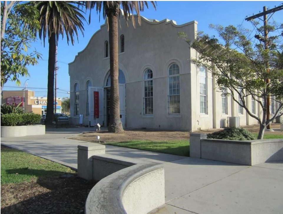
Photo 2 – West Façade and concrete landscaping walls.
