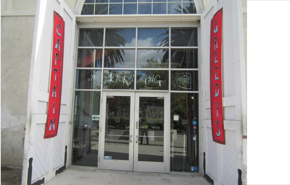
Photo 17 – Wood entry doors and aluminum storefront system at West Façade.
