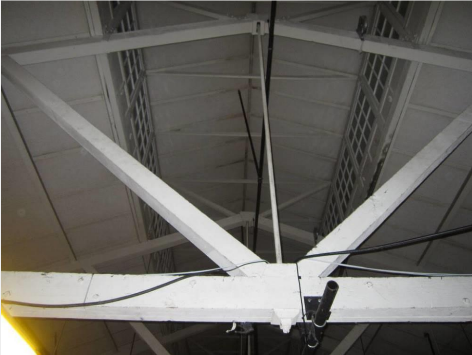
Photo 27 – Existing wood truss at the interior of the building.
