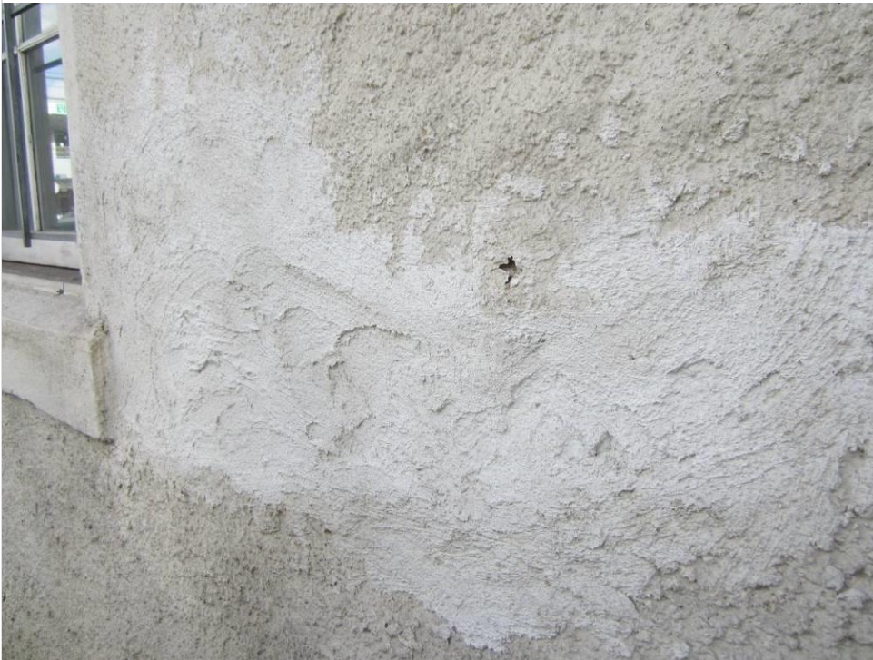
Photo 10 – Previously patched cement plaster wall area.
