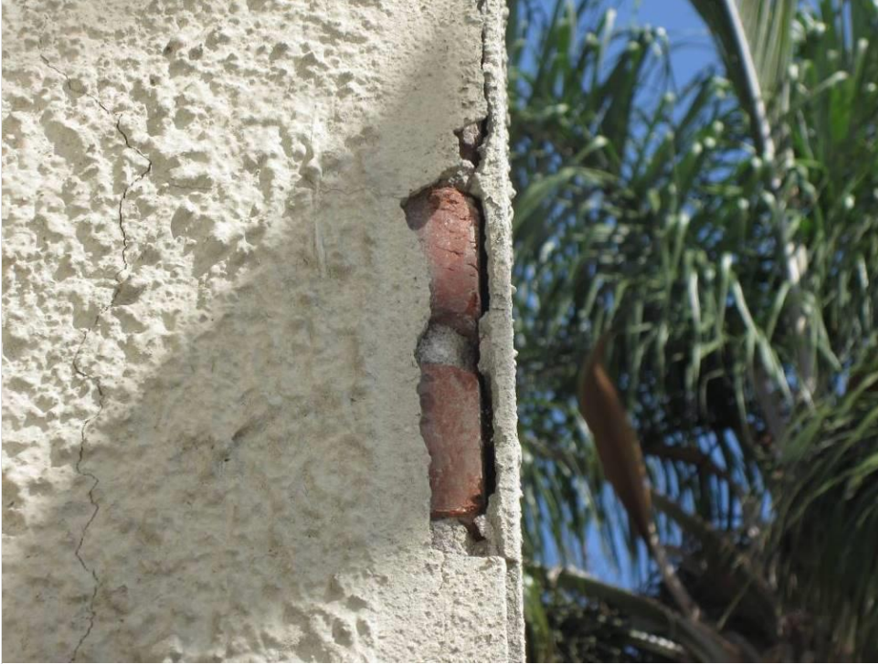
Photo 9 – Exposed brick masonry and mortar joints behind cement plaster.
