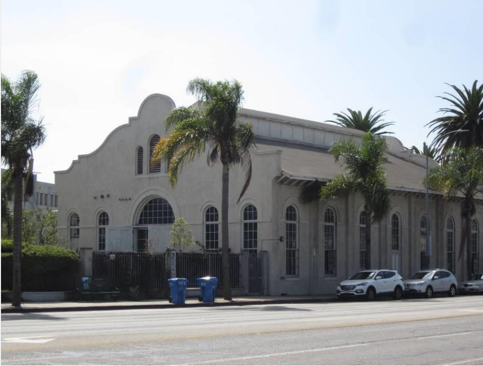
Photo 1 – View of building – East Façade at left and North Façade at right.
