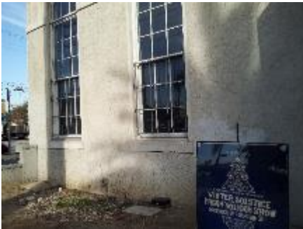
E-31: GFCI outlet on exterior wall not in good working condition
