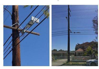
When an applicant can demonstrate that it is i) infeasible to attach their antenna and radio to the top of a utility pole; **and** ii) infeasible to strand mount, **and** iii) infeasible to attach to or replace a nearby streetlight, then the antenna and radio may be placed mid-pole on the utility pole.
