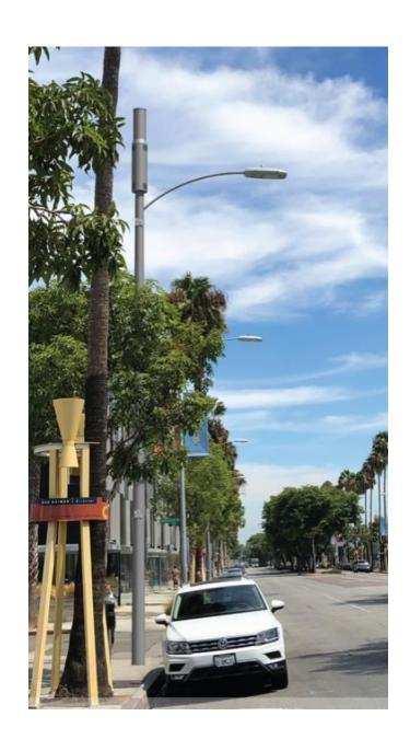
d. Subject to City's approval and execution of a separate agreement, wireless infrastructure providers may remove existing City-owned streetlights and replace them with integrated streetlight poles that contain all of the wireless infrastructure provider's equipment concealed within their interior, so long as the replacement streetlight and pole is substantially similar in type, taper, height, color and texture to the City streetlight being replaced.
