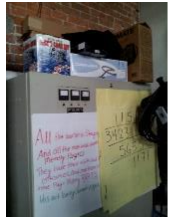
E-10: Inverter not in use
