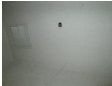
P-3: Existing recessed sprinkler head with no escutcheon
