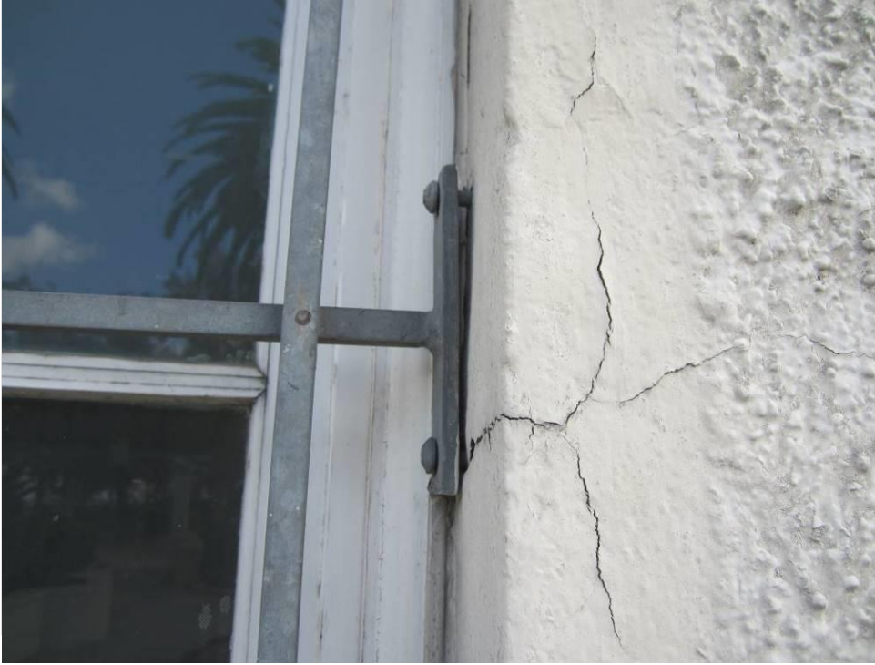
Photo 14 – Wall penetration is not sealed.
