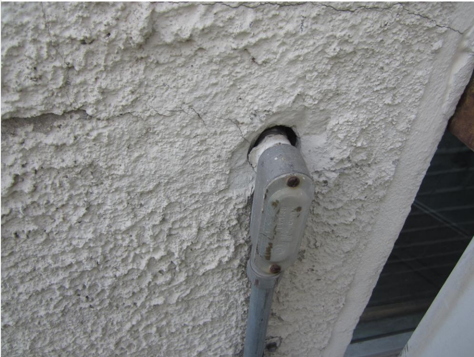
Photo 14 – Wall penetration is not sealed.
