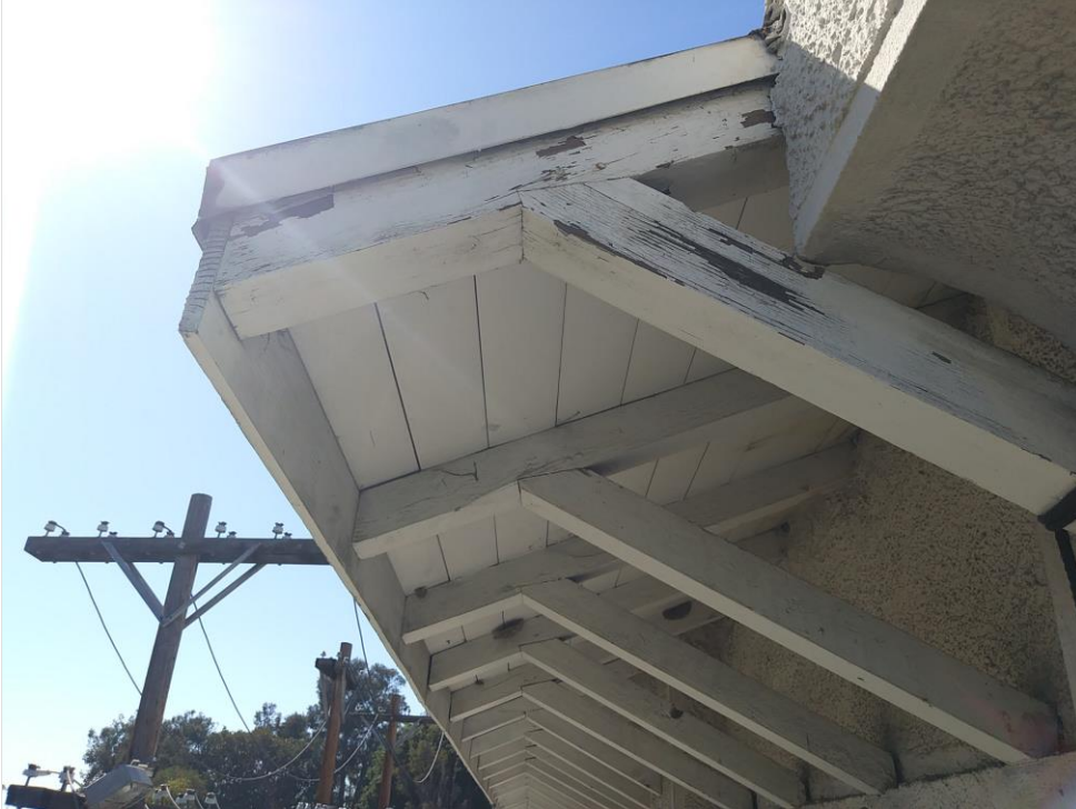
Photo 25 – Paint coating is worn at the edge rafters and diagonal struts that support the roof eave.
