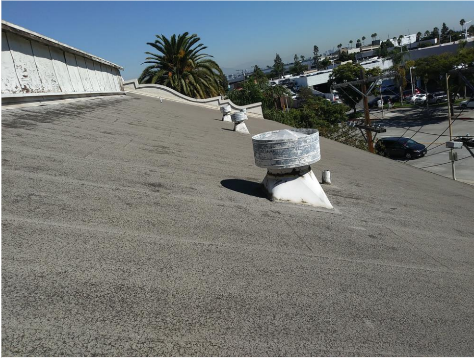
Photo 21 – Existing roofing membrane and vent penetrations.
