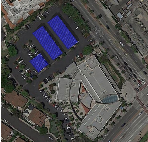
Figure 3. Senior Center 187 kW PV
