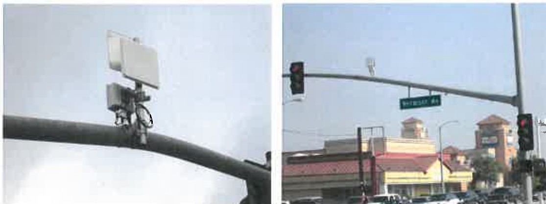
Figure 10 – Typical WLAN Access Point Equipment Installations
