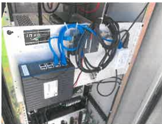
Figure 11 – AP Equipment Panel in Type 332 Traffic Cabinet
