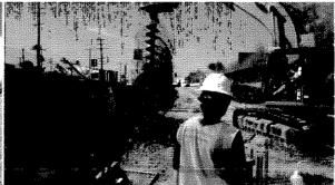
**Challenge:** Beginning of MSE walls construction required constant geotechnical observation during excavation to clearly identify faults, geophysical anomalies and unsuitable soils. These areas were unable to receive the designed loads that require the MSE walls then; recommendation was needed on site to continue the construction process.
