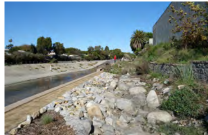
Ballona Creek rain gardens Creek-side rain garden Collects rain water from roofs + parking lots
