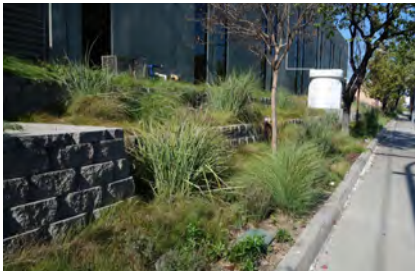
City Maintenance Operations Building “Front yard” rain garden Collects rain water from roof
