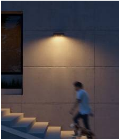
A Wall mounted, low glare, floodlight, illuminating alley entrance
