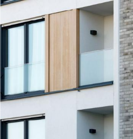
C Unit balcony sconces, providing a subtle glow on ceilings and floors of individual units
