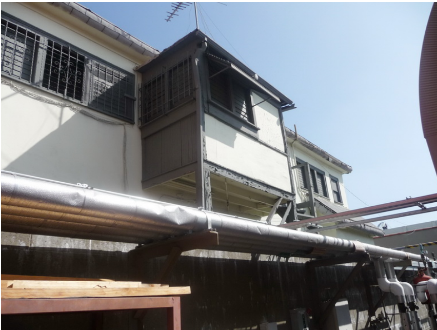
Detail of rear (south) façade, with projecting addition.
