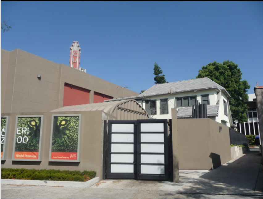
Rear (south) façade of building and rear lot, view facing northwest
