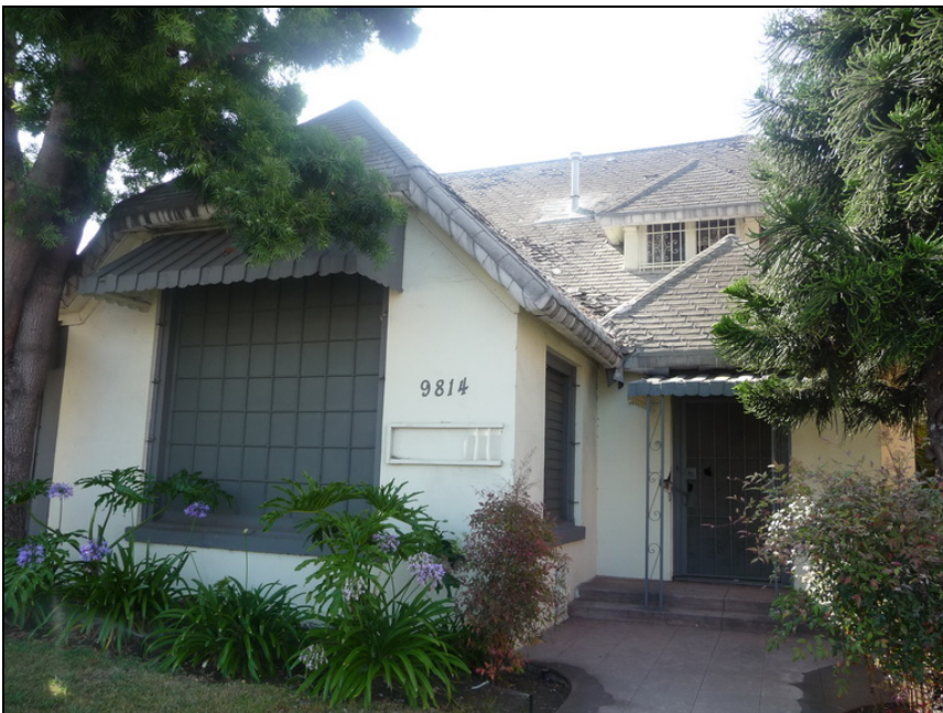
View facing southeast, detail of main façade
