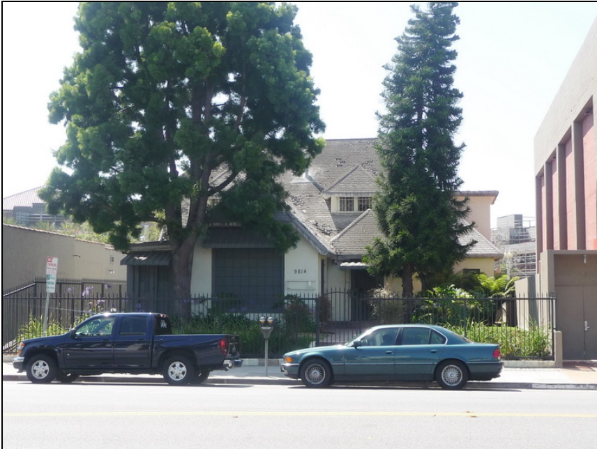
9814 Washington Boulevard, Culver City, view facing southeast
