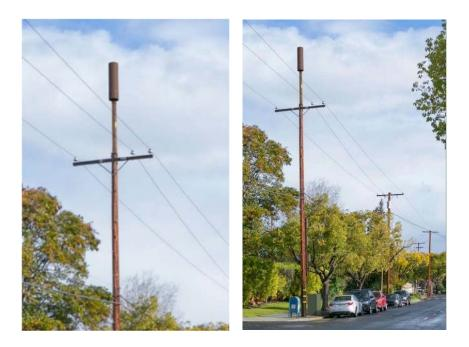
(B) Below is an example of an acceptable radio and antenna strand-mounted on aerial fiber optic cable:
