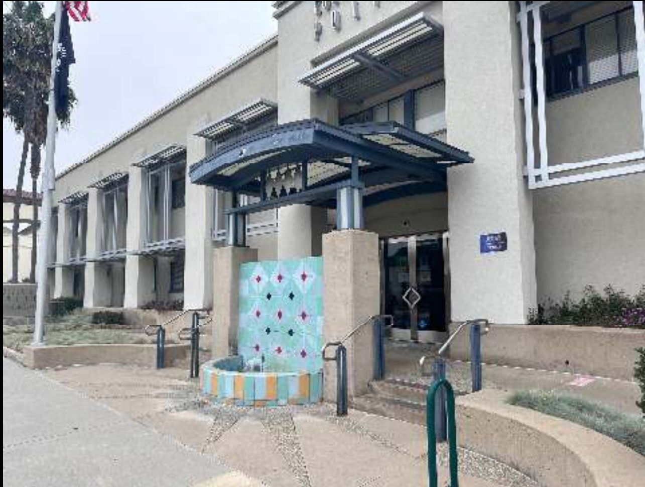
Looking north at the façade of Culver City Police Department.
