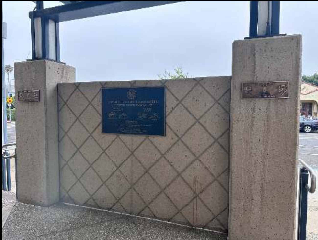
Back concrete wall of Sentry at Culver City Police Department.
