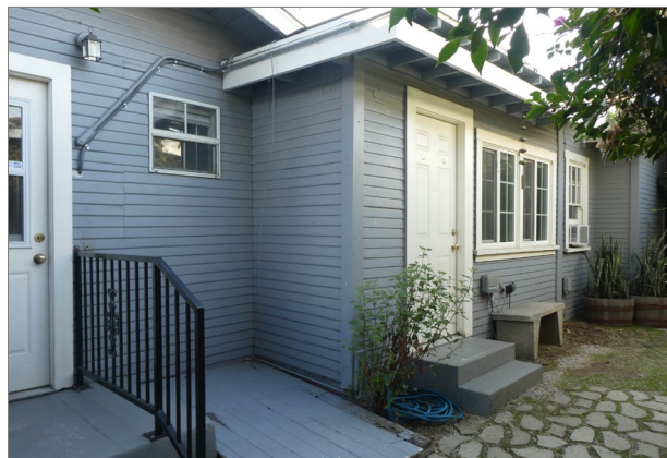
Figure 5: Rear elevation, view looking west. Source: GPA, December 2019.
