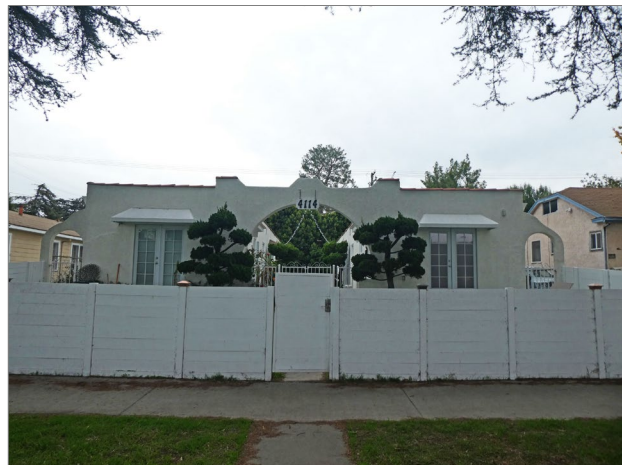
Figure 17: 4114 Lafayette Place, view looking northeast. Source: GPA, December 2019.
