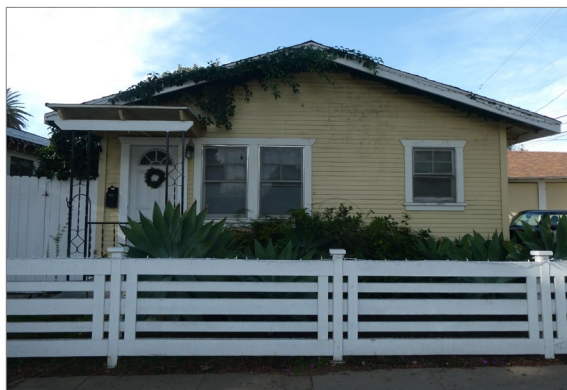
Figure 7: Façade, view looking west. Source: GPA, December 2019.
