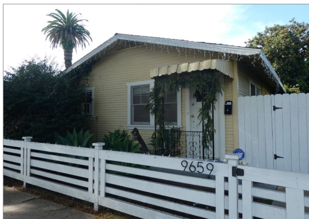
Figure 6: Façade, view looking west. Source: GPA, December 2019.
