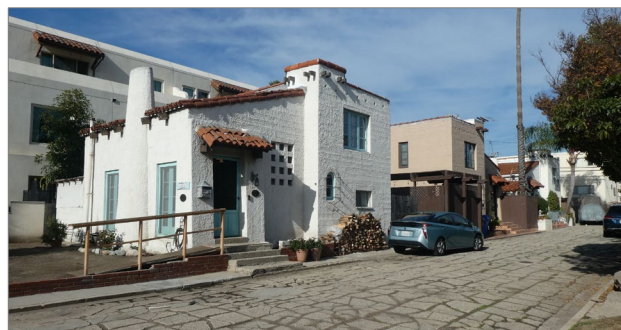
Figure 15: 4052A-4052C Lafayette Place, view looking north. Source: GPA, December 2019.
