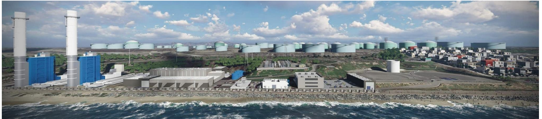
North Site, ESGS
