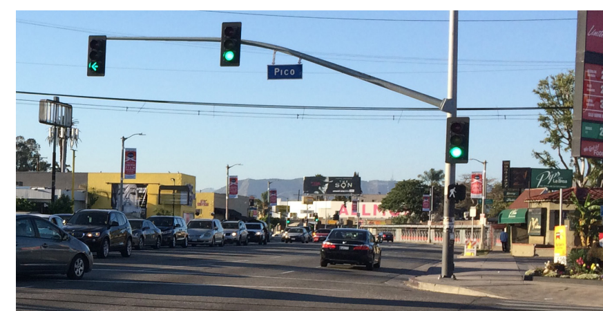
Protected left turn phases reduce conflict between turning vehicles and users of all modes.
