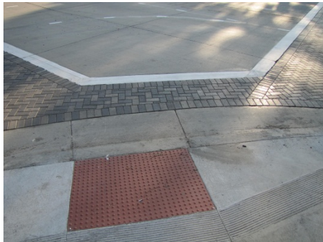
Detail: Curb ramp installation.
