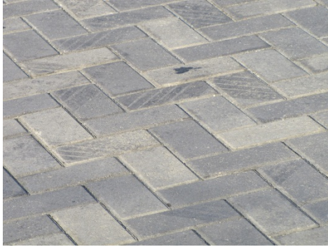
Detail: Herringbone paver pattern.
