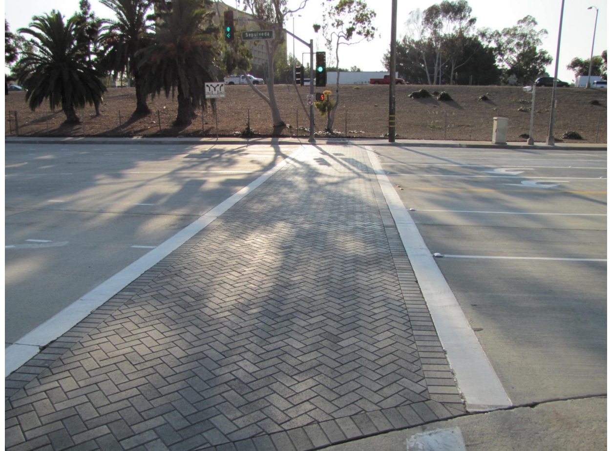
Completed Inter-locking Concrete Paver installation.
