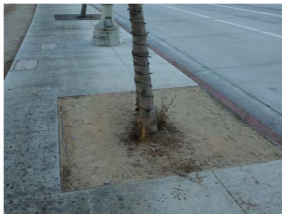
Tree grate replaced with decomposed granite Culver Blvd near Downtown
