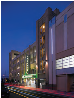
Civic Center Parking Structure, Alameda, CA
