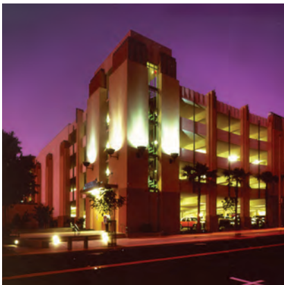
Downtown Parking Structure, Ventura, CA
