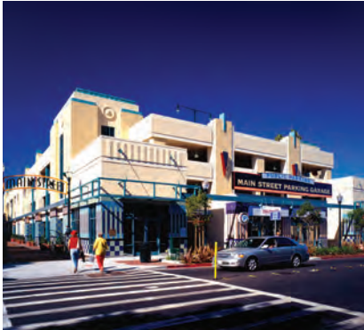
Main Street Parking Structure, San Mateo, CA
