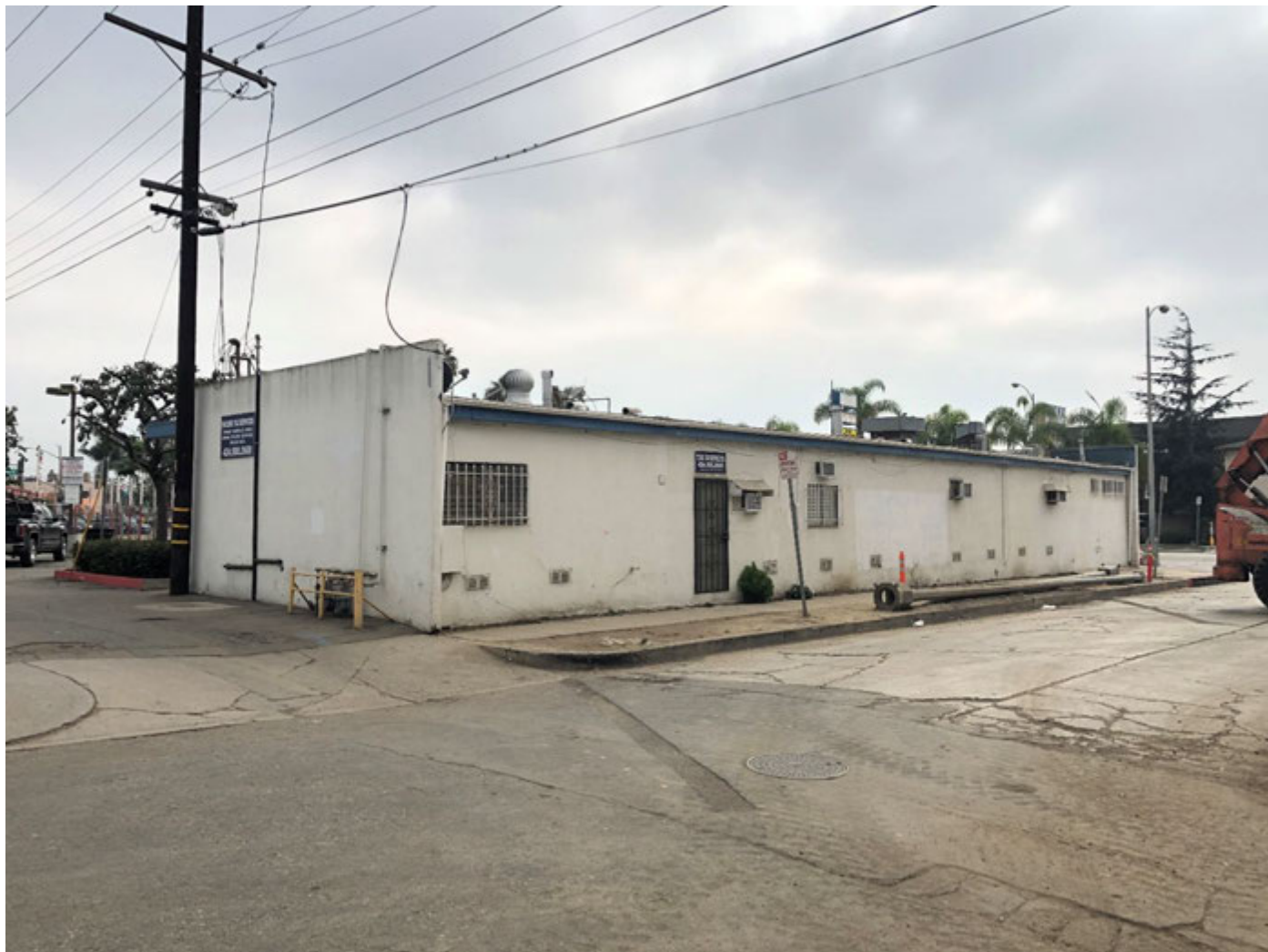
North and west elevations, facing southeast
