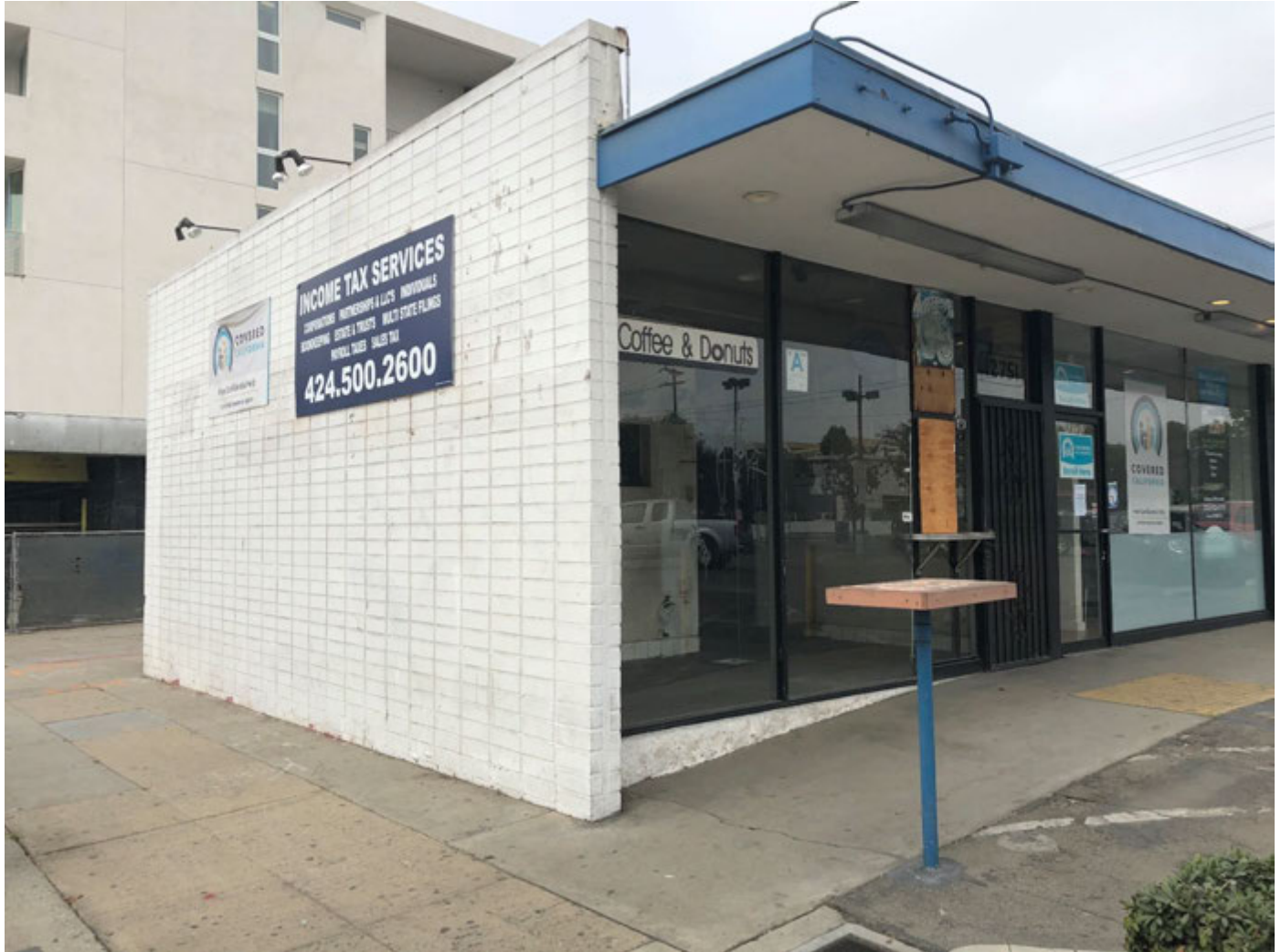
South elevation, facing northwest
