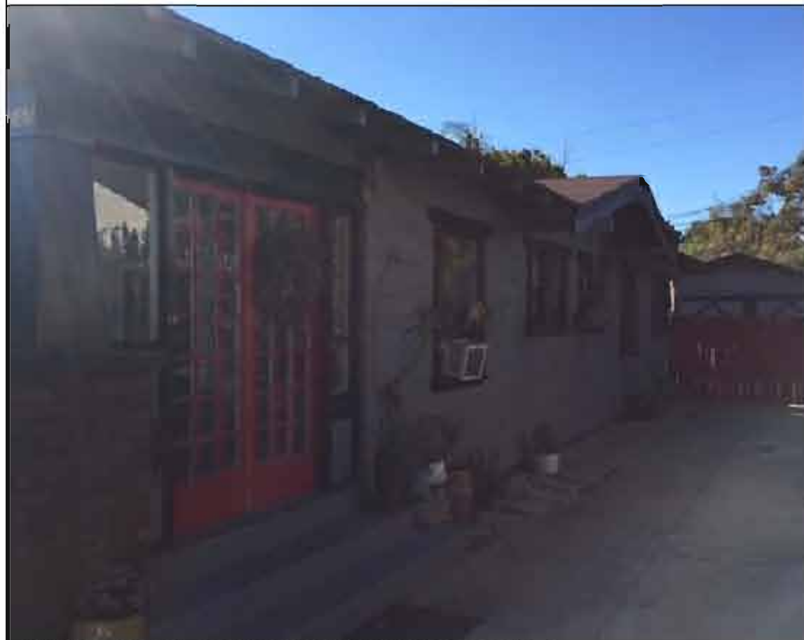
(iv) OPENINGS ON SOUTH ADJACENT PROPERTY
