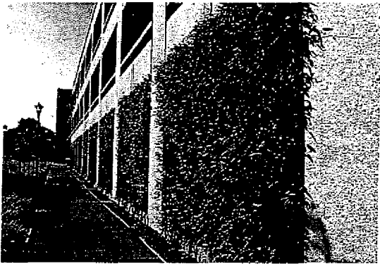
Parking Structure - Palo Alto, CA
