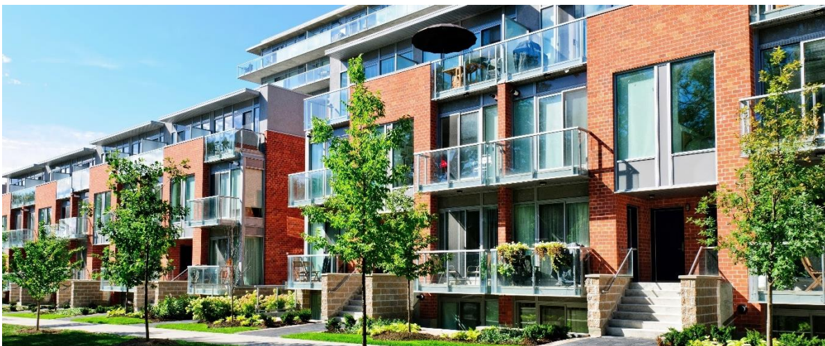
Above: Stoop frontages create an active and welcoming streetscape.
