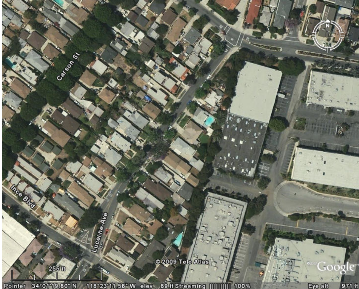
FIGURE 2, AERIAL VIEW OF THE 9000 BLOCK OF LUCERNE AVENUE
