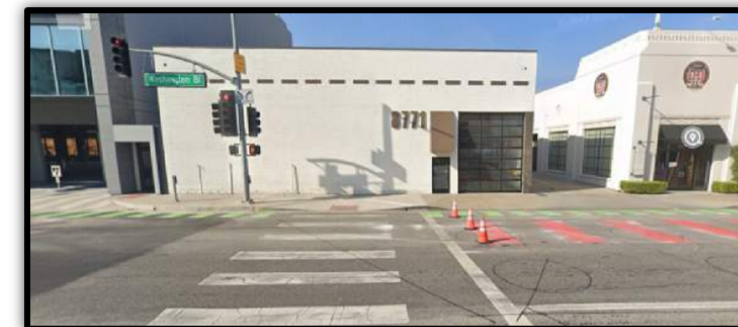
Washington Blvd ( Phase 1 - Shoring )
