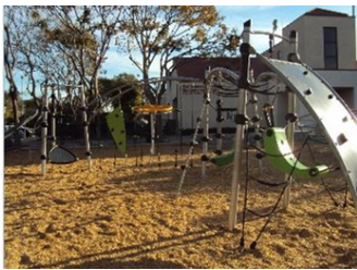
Playground Equipment Repair at Parks
