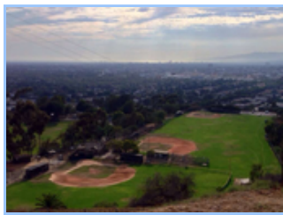
Culver City Park Baseball Fields Repairs
