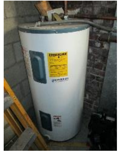
P-2: Existing water heater will have seismic bracing
