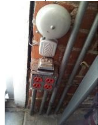
E-6: Fire alarm sprinkler bell and receptacle outlet
