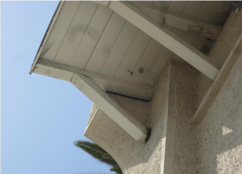
Photo 26 – Diagonal wood strut needs to be reattached to the wall. Gap between the wall and roof interface needs to be sealed.
