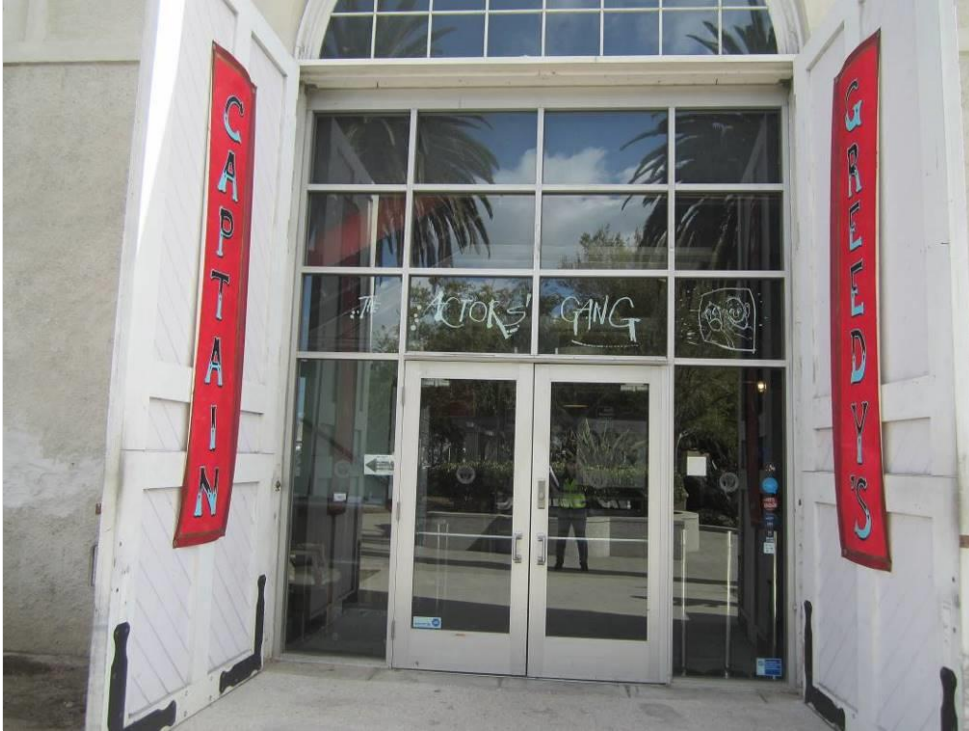
Photo 17 – Wood entry doors and aluminum storefront system at West Façade.
