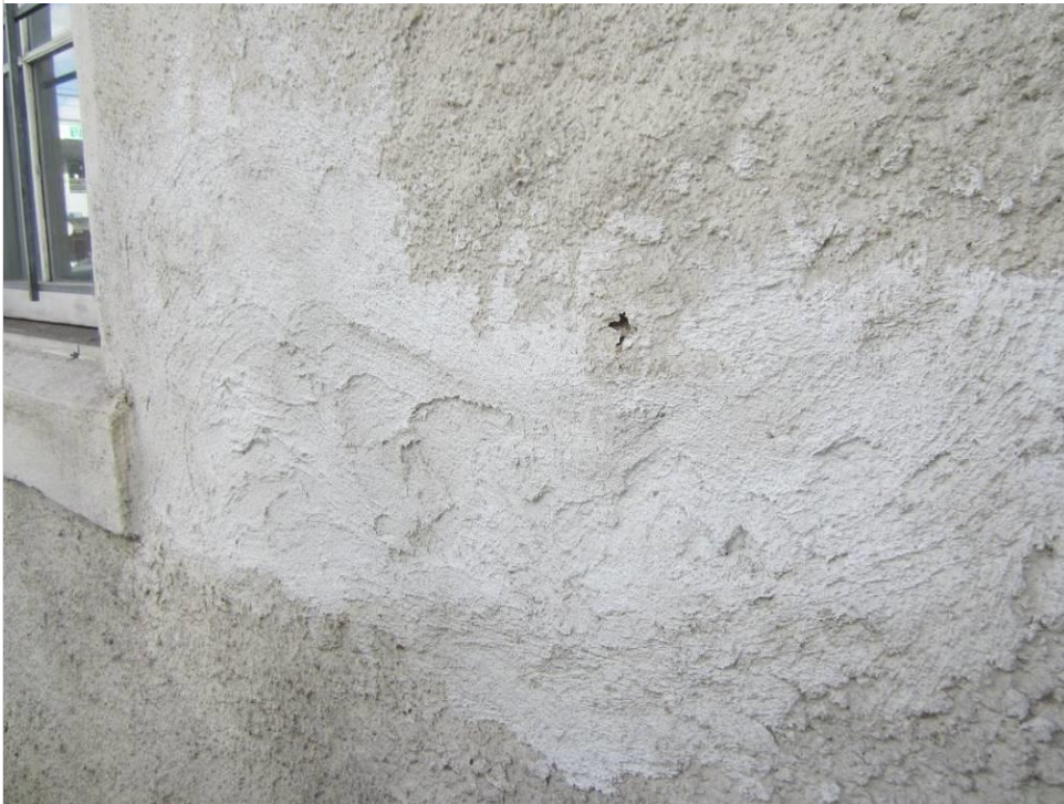
Photo 10 – Previously patched cement plaster wall area.
