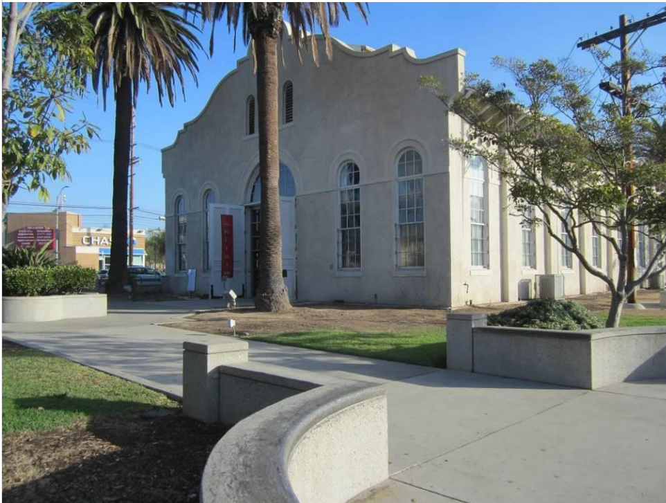
Photo 2 – West Façade and concrete landscaping walls.
