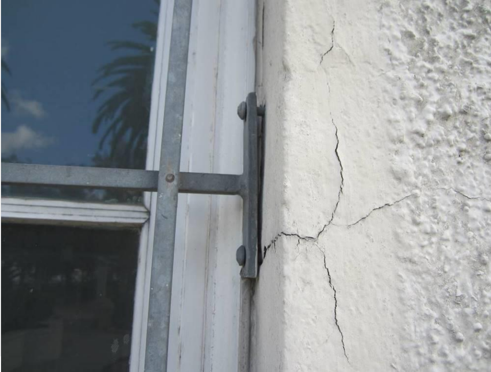
Photo 14 – Wall penetration is not sealed.
