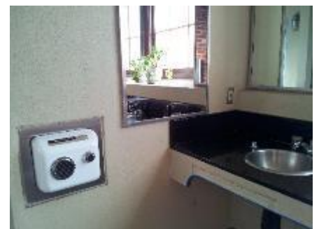
E-8: Hand dryer and GFCI in men's restroom
