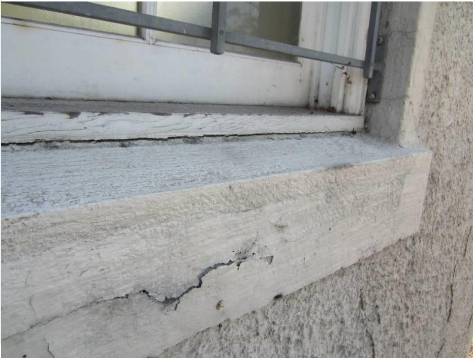
Photo 16 – Wood window sill and concrete ledger with crack in paint coating. Note that the joint between the wood sill and ledger is not sealed.
