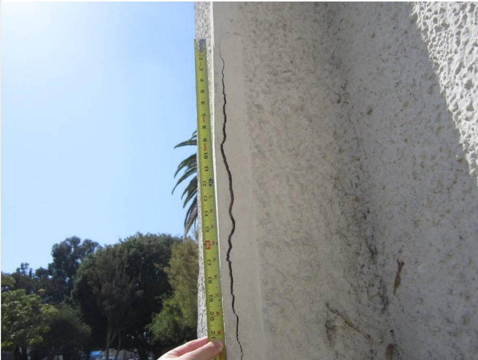
Photo 6 – Vertical crack in existing cement plaster wall.
