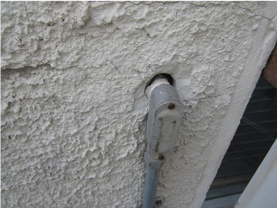
Photo 14 – Wall penetration is not sealed.
