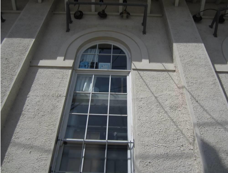
Photo 6 – Vertical crack in existing cement plaster wall.
