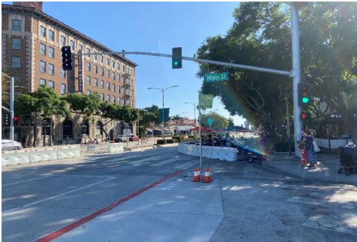
Culver Boulevard & Main Street - Westbound - Looking West
