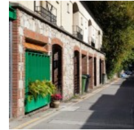
Rehab Story: From Garage to Garden for a Dublin Carriage House
