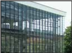
③ Steel Framed Curtain Wall
