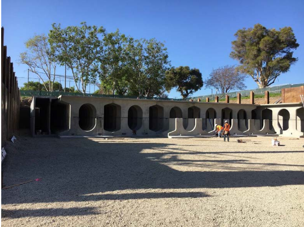
Figure 3-4. Typical Concrete Storage System
