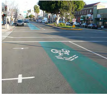
Shared Lane pavement marking with colored Green Lane on 2 nd Street in Long Beach, CA.
