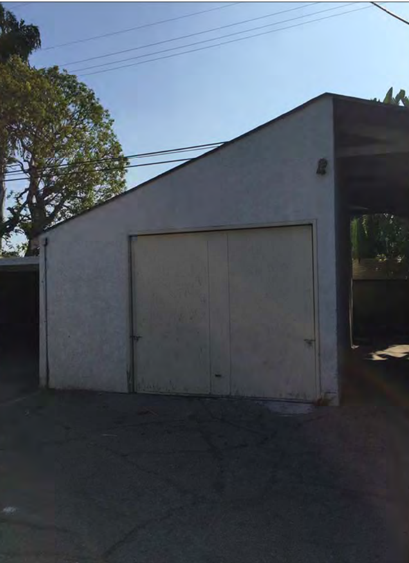
EXISTING BUILDING PHOTOS : Rear Carport
