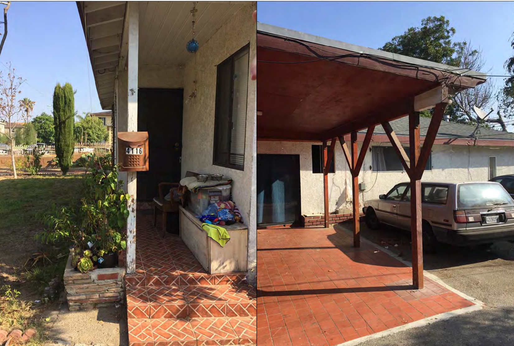
EXISTING BUILDING PHOTOS : South Facade
