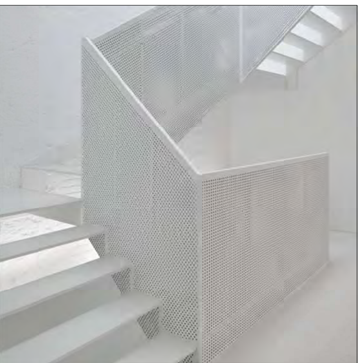
INTERNAL STAIRS WHITE POWDER COATED PERFORATED METAL BALUSTRADE WITH SOTNE TILE THREADS
