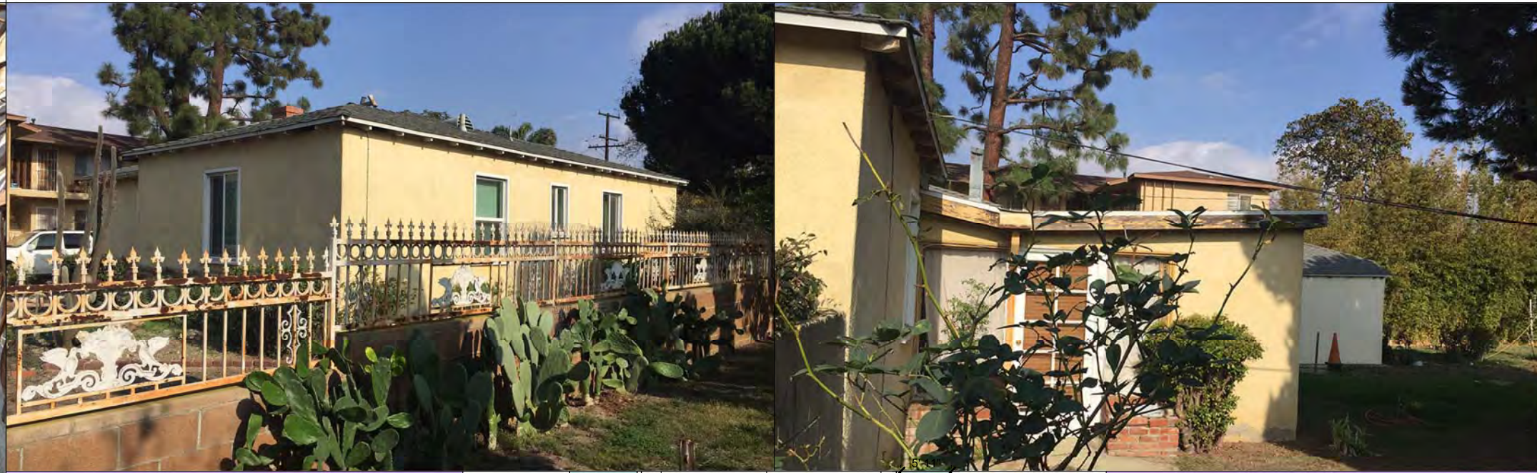
EXISTING SITE PHOTOS : North Adjacent Property
