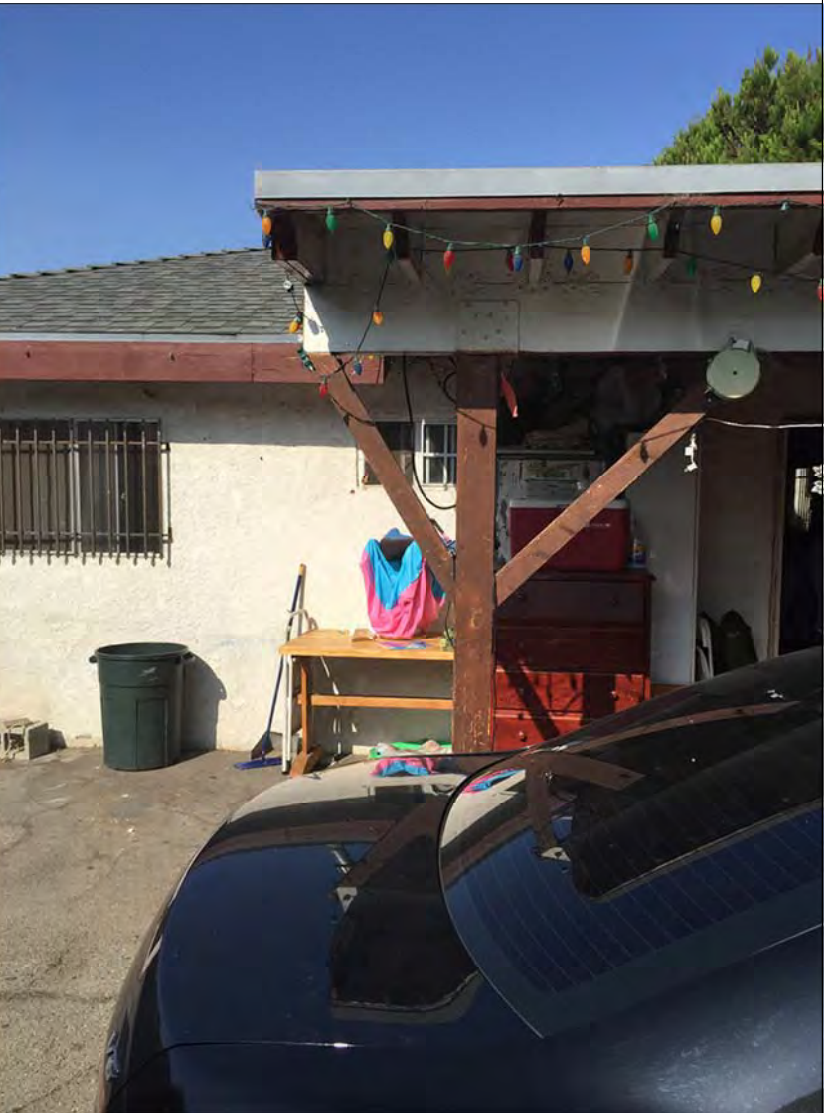
EXISTING BUILDING PHOTOS : East Facade
