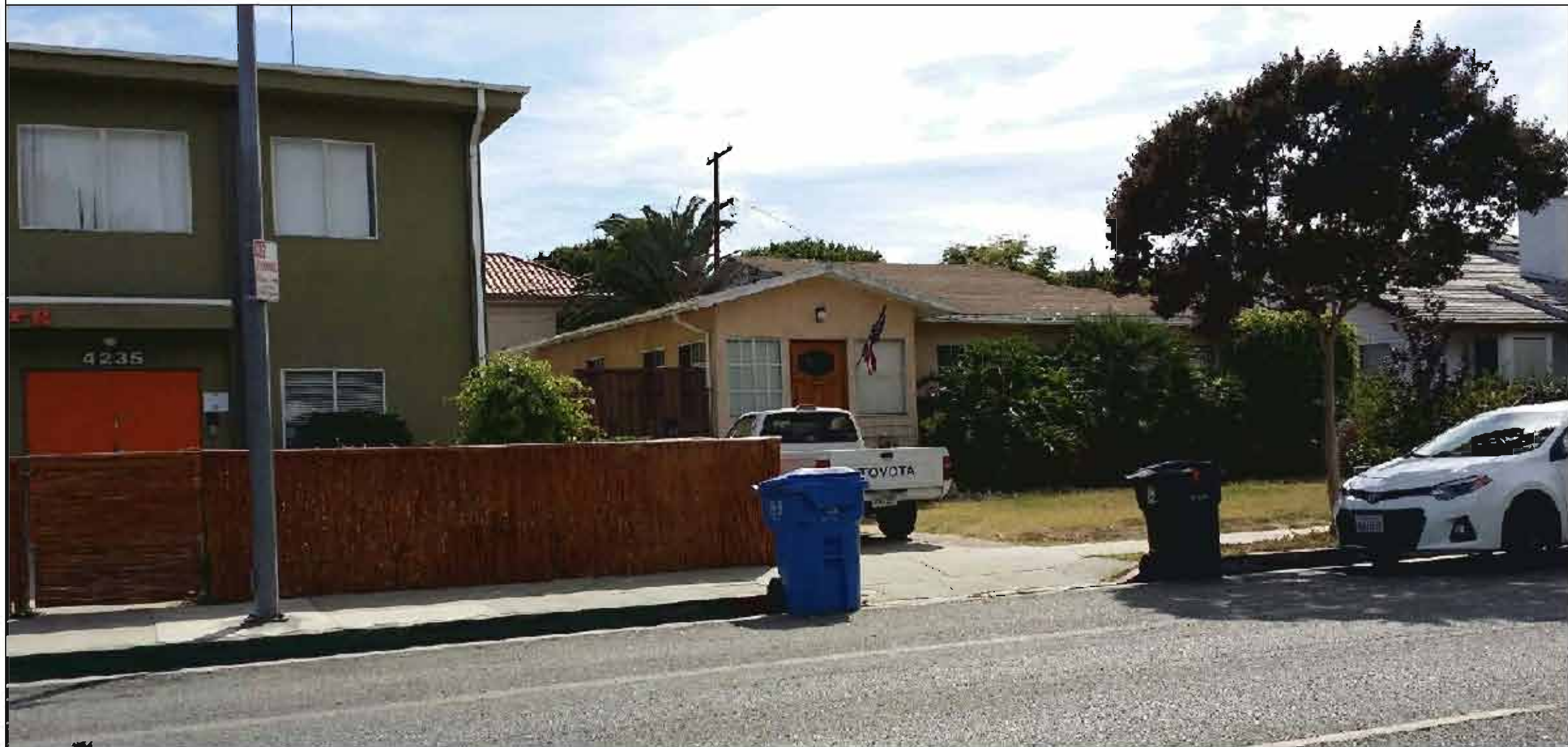
(vi) NORTH ADJACENT PROPERTY ON DUQUESNE
