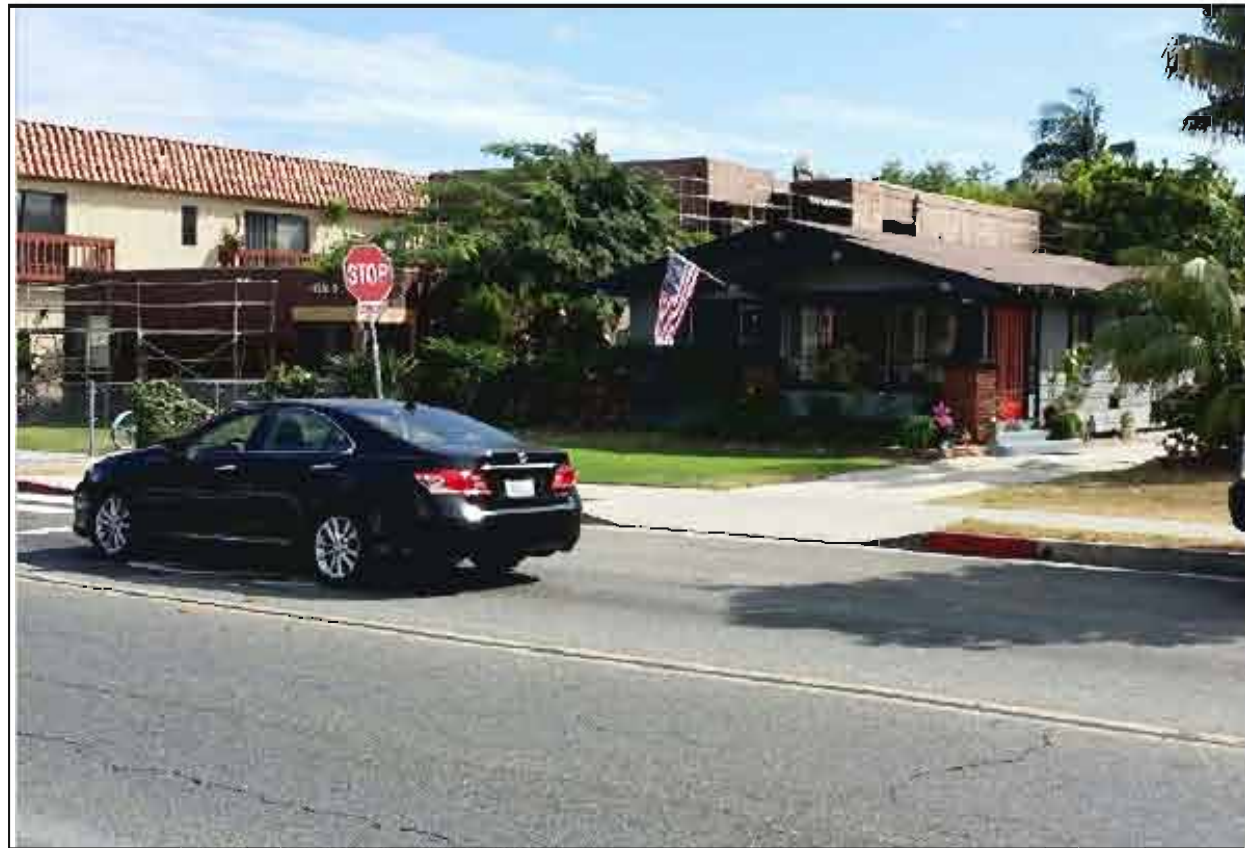
(i) SOUTH ADJACENT PROPERTY
