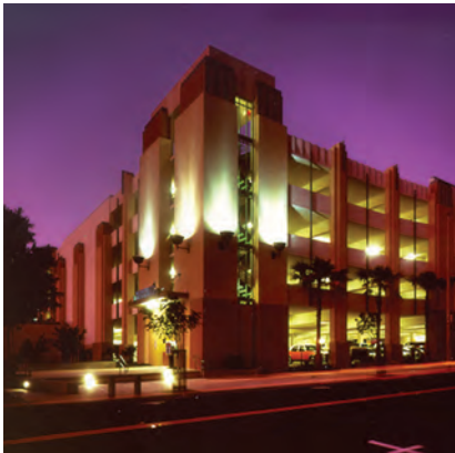
Downtown Parking Structure, Ventura, CA
