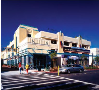
Main Street Parking Structure, San Mateo, CA
