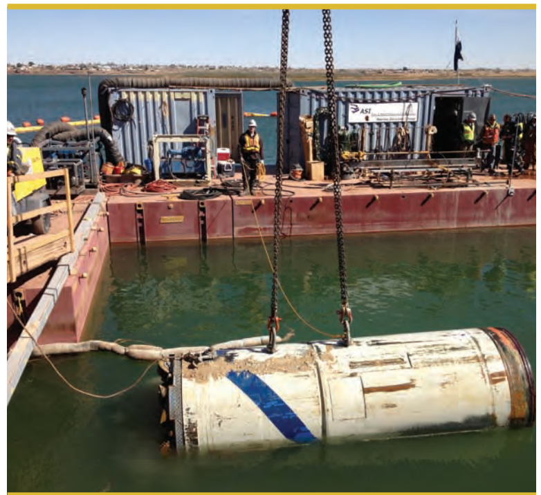
THE MTBM WAS RECOVERED AT 50-FT DEPTHS BY DRIVERS WHO CONNECTED IT TO A SLING, THEN HOISTED IT TO THE SURFACE VIA CRANE.
