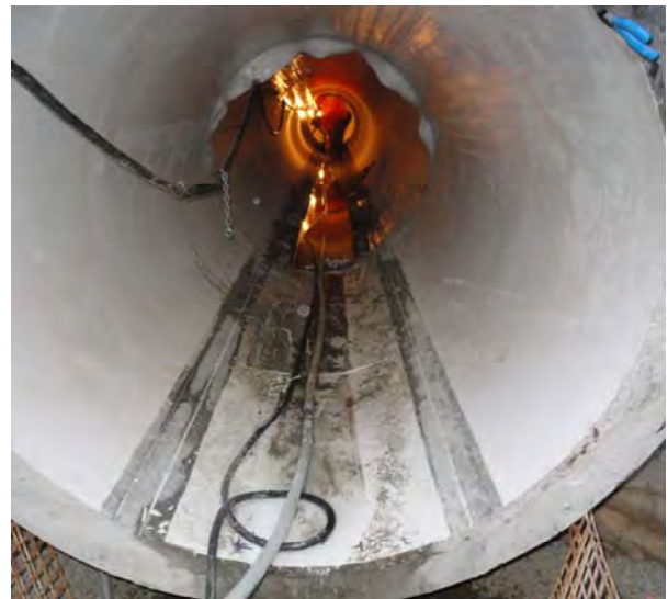
Recoverable Jacking Can with over 600 tons of thrust capacity
