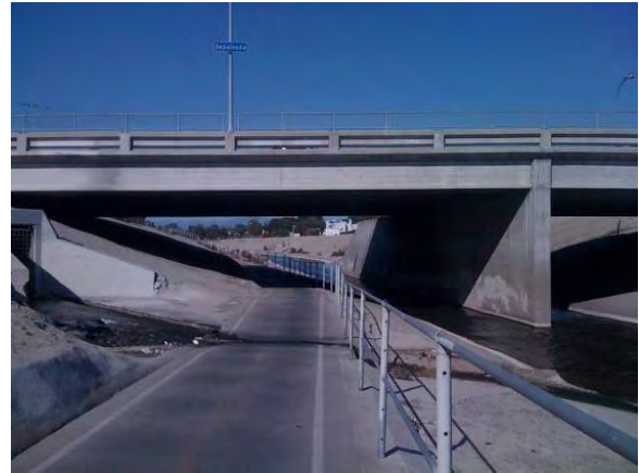
Ballona Creek Path at Sepulveda Boulevard
