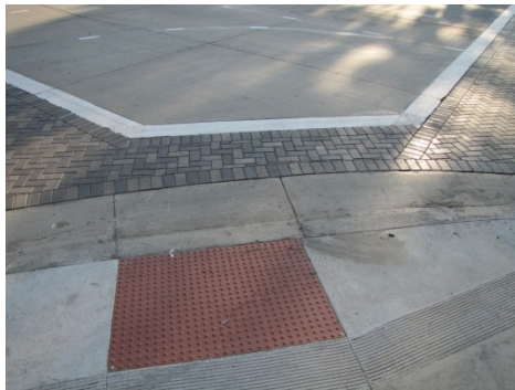
Detail: Curb ramp installation.
