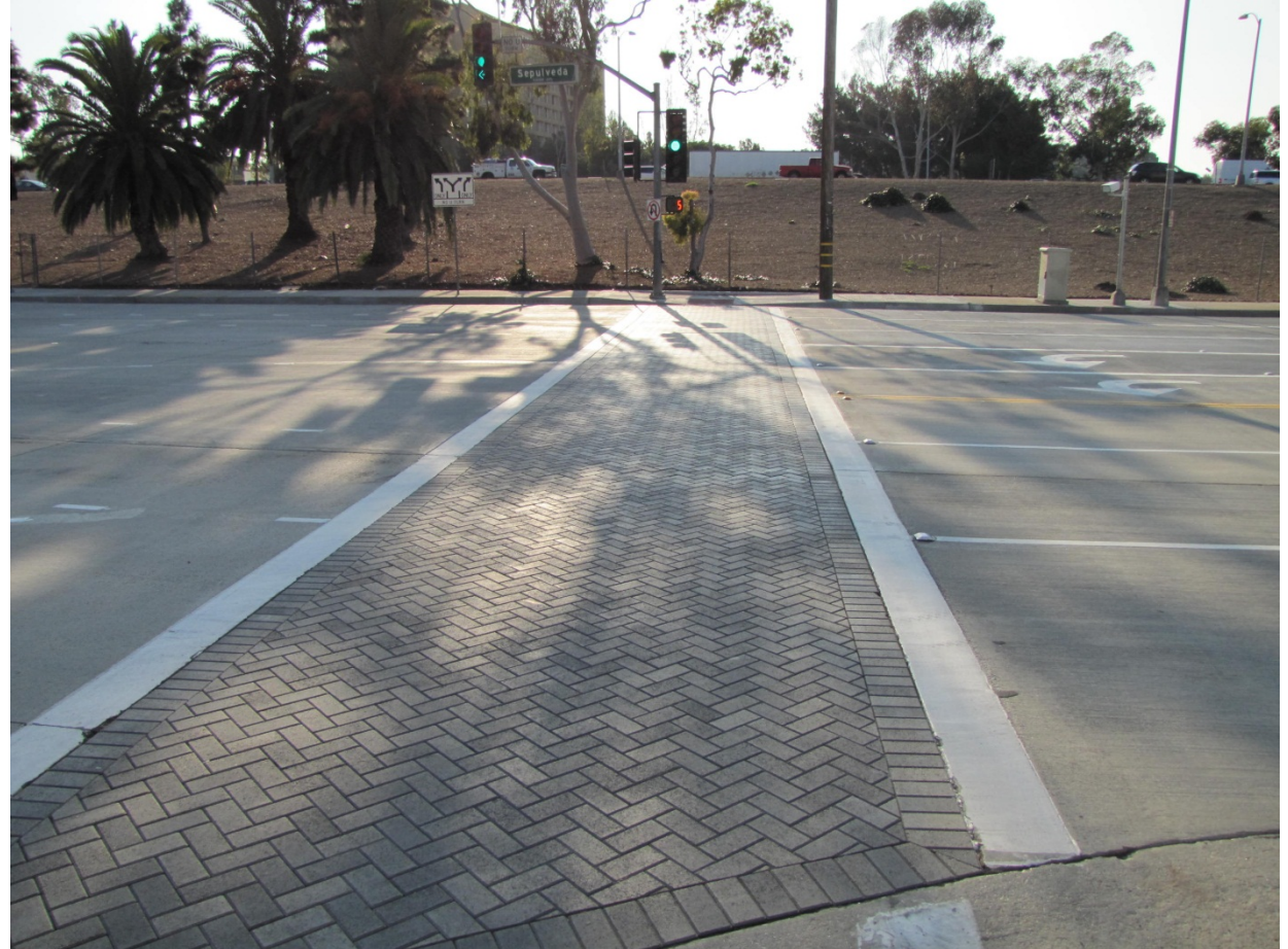
Completed Inter-locking Concrete Paver installation.
