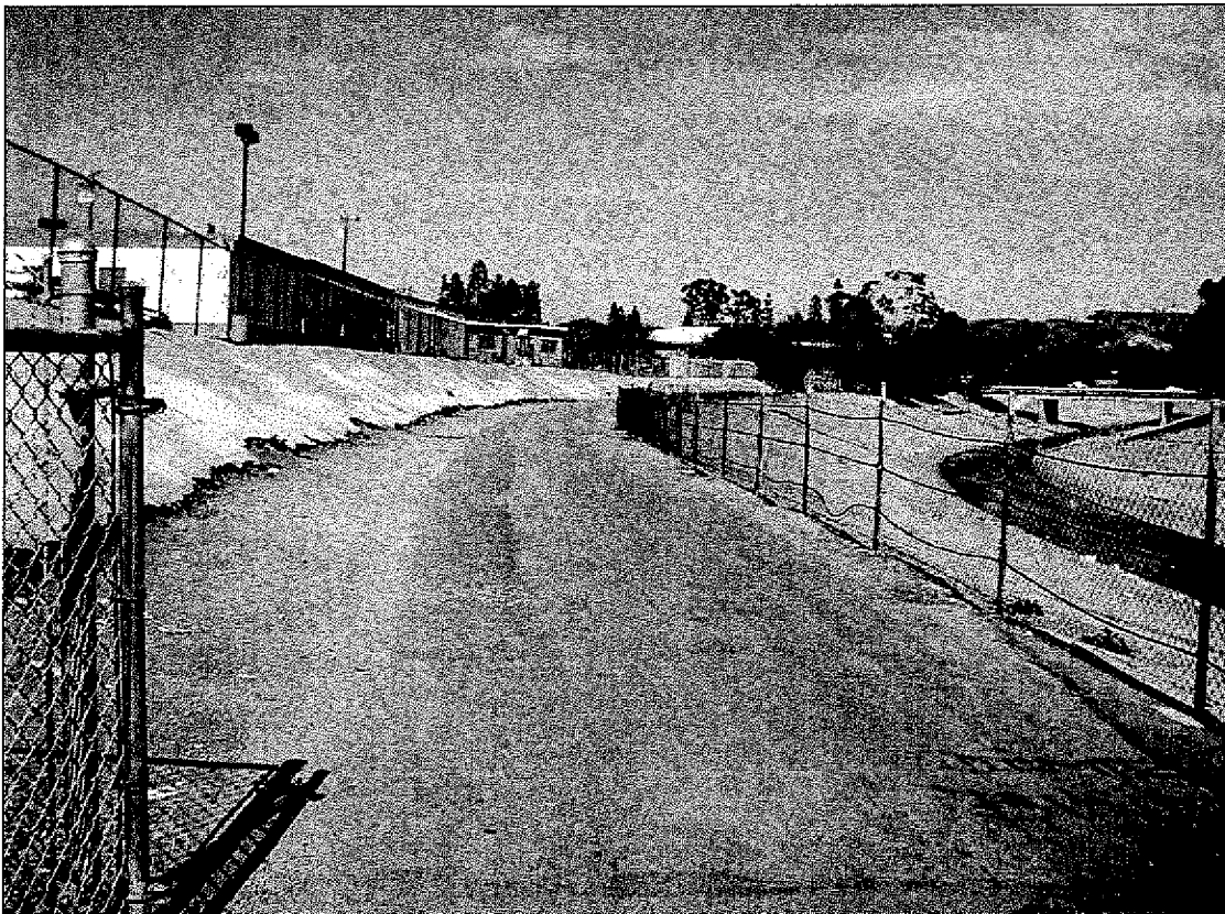
Exhibit 7: Existing Path Condition Photo
