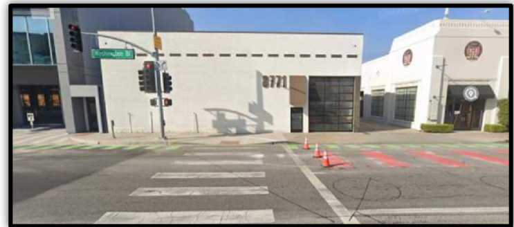
Washington Blvd ( Phase 1 - Shoring )
