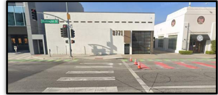
Washington Blvd ( Phase 1 - Excavation )
