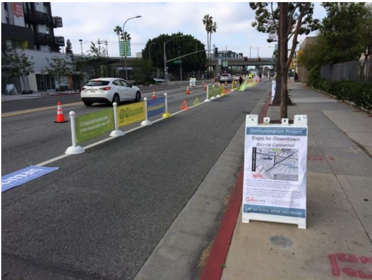
Photo from March 26th Demonstration Project
