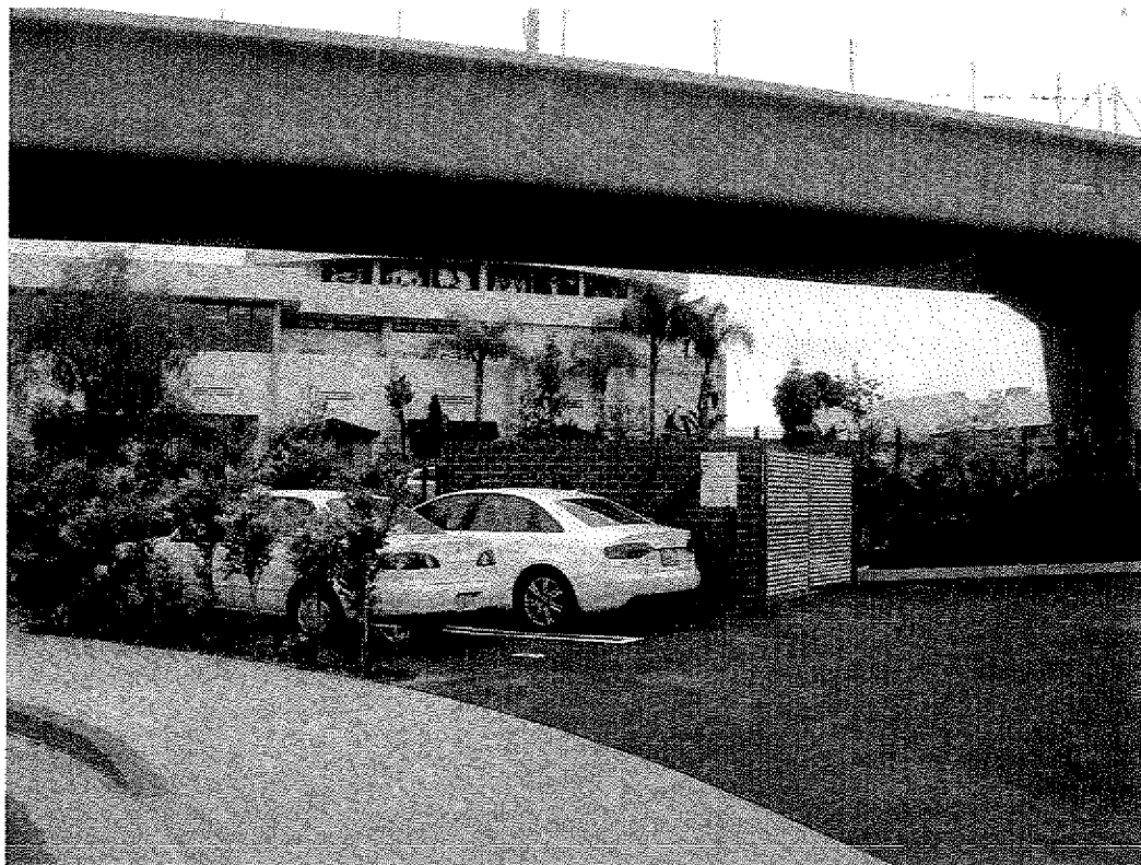
View of subject from Wesley Street facing south.
