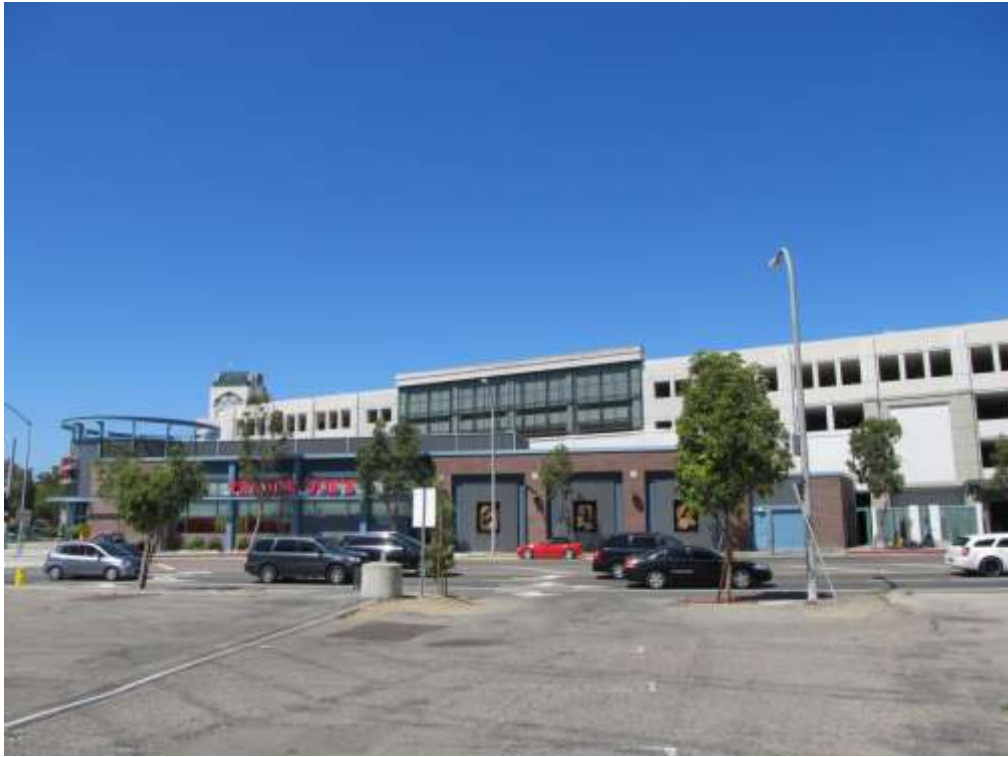
View east from the subject property across Washington Blvd. to the City-owned parking structure.
