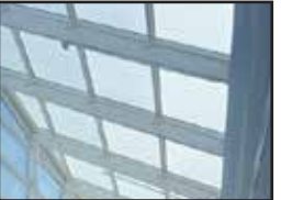
③ Glass Skylight
