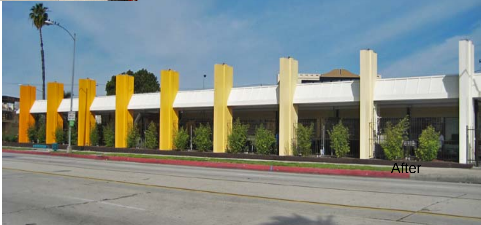
Commercial Façade Rehabilitation
