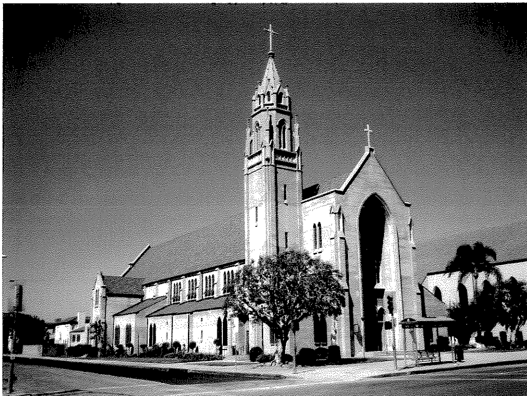
Church Main Entrance
