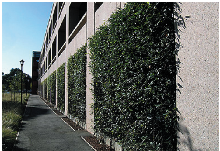
Parking Structure - Palo Alto, CA
