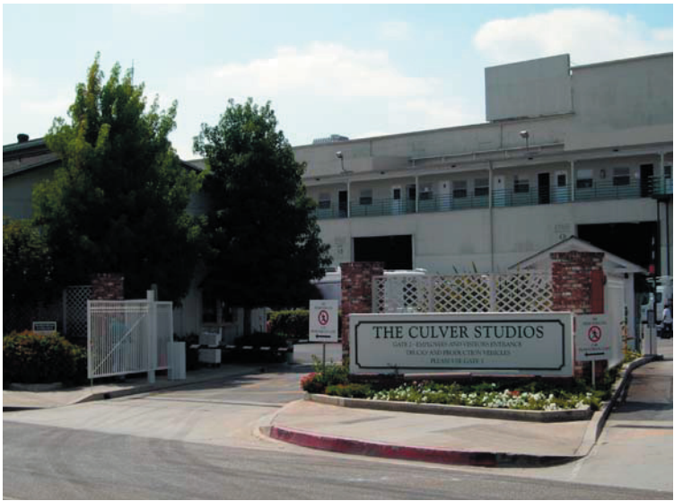
Existing landscaping at Gate 2
