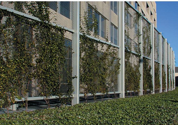
Parking Structure - Tustin, CA
