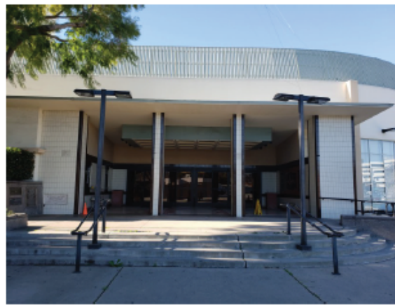
2 EXISTING SITE CONDITION SCALE: NTS
