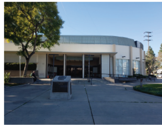
3 EXISTING SITE CONDITION SCALE: NTS
