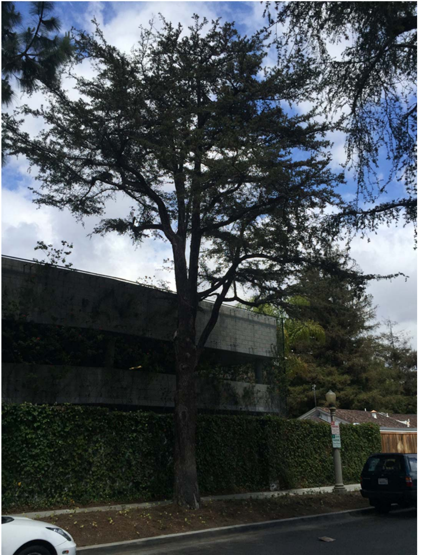
Photo showing decay at the base of the 5 th tree going from north to south
