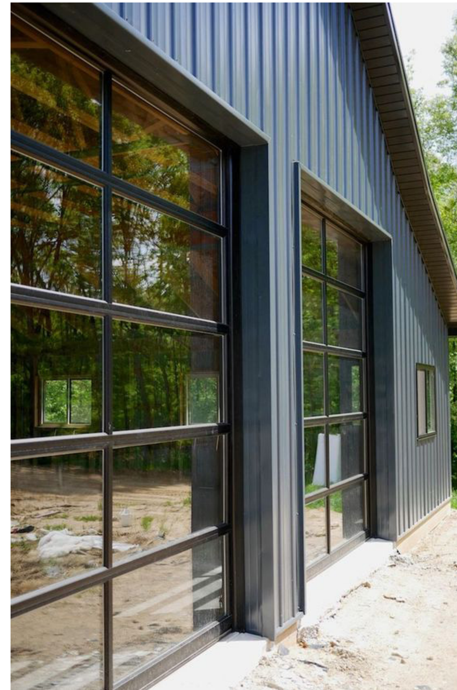
ROLL UP DOORS _ Color to Match Development Storefronts (70% Kynar to match PPG CL3176N RACCOON)
