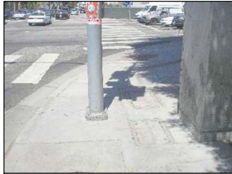
EXISTING 3' CLEARANCE BETWEEN TRAFFIC SIGNAL POLE AND CONTROLLER CABINET. RECOMMENDED TRAFFIC SIGNAL MODIFICATION TO INCREASE CLEARANCE.
