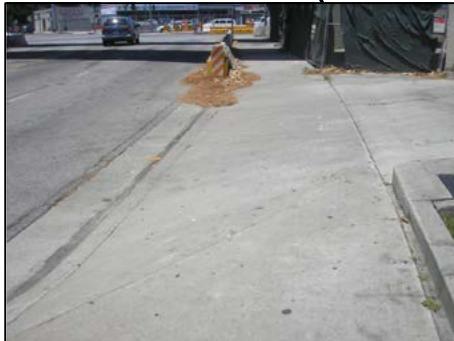
EXISTING DRIVEWAY DOES NOT MEET ADA REQUIREMENTS. RECOMMEND RECONSTRUCTION OF DRIVEWAY TO MEET CURRENT STANDARDS
