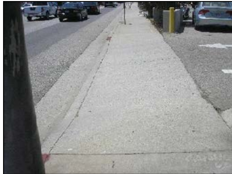
RECONSTRUCT DRIVEWAYS TO MEET ADA REQUIREMENTS.
