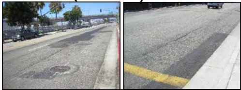
DAMAGED PAVEMENT. REMOVE AND REPAIR.
