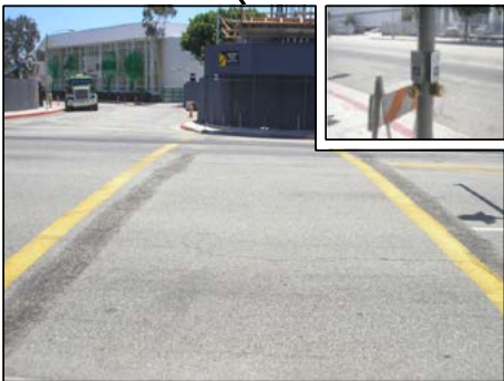
UPGRADE CROSSWALK TO CONTINENTAL CROSSWALK OR WITH DECORATIVE PAVERS. UPGRADE ALL PEDESTRIAN PUSH BUTTONS TO CITY APPROVED APS UNITS. TYPICAL FOR ALL PPB'S AT THIS LOCATION.
