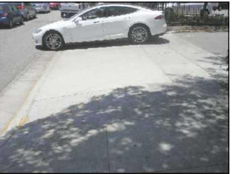
PEDESTRIAN PATH AT BACK OF DRIVEWAY IS 3'. RECOMMEND TO RECONSTRUCT DRIVEWAY TO ACCOMPLISH A 4' MINIMUM PEDESRIAN PATH AT 2%.
