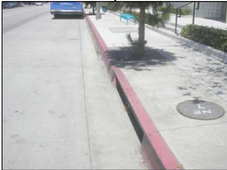
EX. CATCH BASIN. INSTALL CITY APPROVED CATCH BASIN SCREEN AND/OR DEBRIS COLLECTOR (BMP). OPPORTUNITY TO REMOVE ADJACENT TREE & REPLACE WITH STORM WATER BIORETENTION FILTRATION SYSTEM/TREE WELL (LID)
