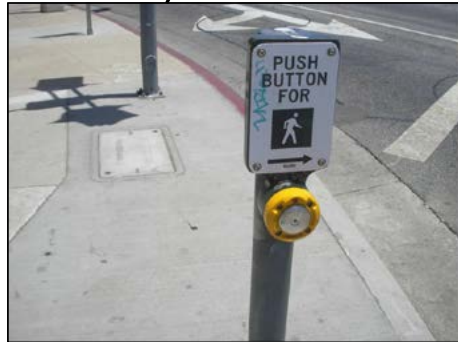
RECOMMEND TO UPGRADE ALL PEDESTRAIN PUSH BUTTONS TO CITY APPROVED APS UNITS. TYPICAL FOR ALL PPB'S AT THIS INTERSECTION.
