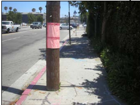
INSTALL CONCRETE BUS PAD.
