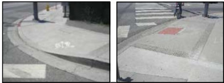
EXISTING RAMP DOES NOT MEET ADA REQUIREMENTS. RECONSTRUCT RAMP TO MEET ADA REQUIREMENTS.
