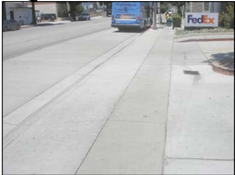
EXISTING DRIVEWAY HAS 3' PEDESTRIAN PATH. RECOMMEND RECONSTRUCTION OF DRIVEWAY WITH A MINIMUM 4' PEDESTRIAN PATH.
