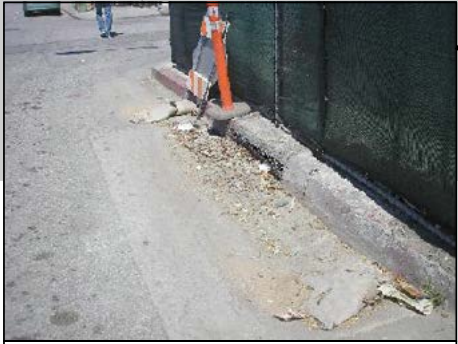
FUTURE RECONSTRUCTED CATCH BASIN. INSTALL CITY APPROVED CATCH BASIN SCREEN AND/OR DEBRIS COLLECTOR (BMP).
