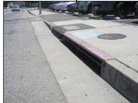
EX. CATCH BASIN. INSTALL CITY APPROVED CATCH BASIN SCREEN AND/OR DEBRIS COLLECTOR (BMP).
