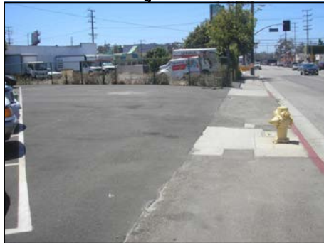
REMOVE AND RECONSTRUCT CURB, GUTTER, AND SIDEWALK AS NEEDED. OPPORTUNITY TO ACQUIRE UNUSED AREA FOR LANDSCAPING AND/OR LID FEATURES.
